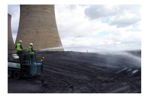
Dustbuster 2 is an environmentally safe, powerful polymer emulsion that produces highly effective control of dust and erosion. It provides superior bonding, cohesion and the ability to penetrate, saturate and bond surface dust and aggregate together. The result is a hard, dust free water resistant resilient surface.
